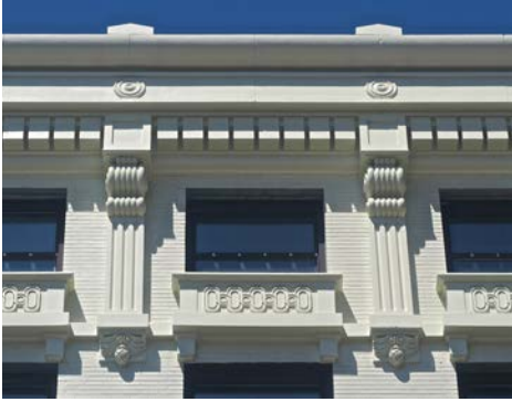
Above: details of the new lightweight cornice and painted brick.
