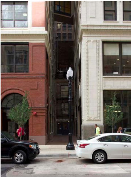
Below: facing north into Pickwick Alley situated between the Gibbons (left) and Steger (right) buildings.
